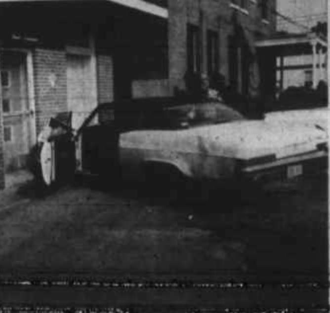
The car above was heavily damaged and two occupants received minor injuries when it came to a sudden stop as it hit the Texas Eastern Co. brick office building on FM 102 last Wednesday afternoon.
